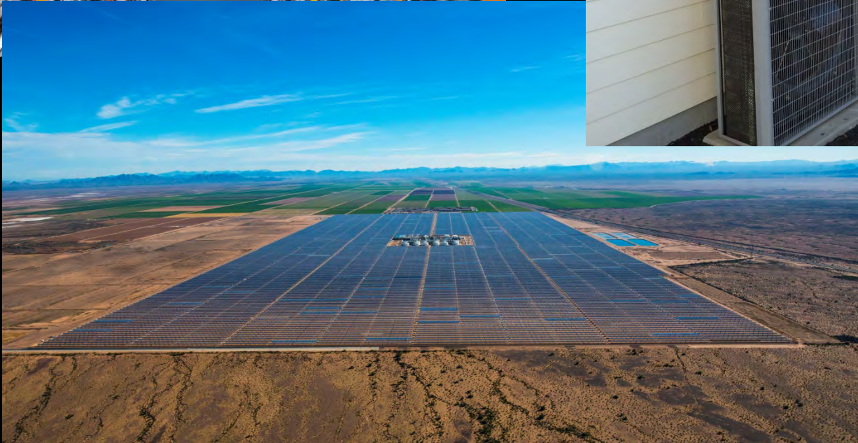
Abengoa Solana Solar Thermal with Storage
